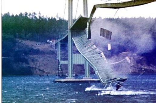
Figure 5.1: Collapse of the Tacoma Narrows Bridge.
